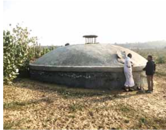
Cluster storage tank, Ramzan ki Gafan, Barmer
